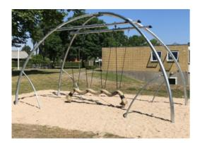
The steel pipes are hot dip galvanised inside and outside with lead free zinc. The galvanisation has excellent corrosion resistance in outside environments and requires low maintenance.
