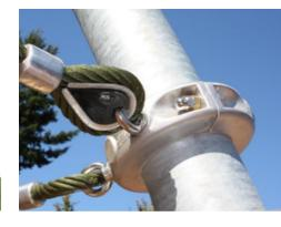
Corocord aluminium clamps are used as connectors between steel posts and rope. Two aluminium castings are bolted together. The height of the clamps is thus variable.
