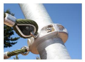
Corocord aluminum clamps are used as connectors between steel posts and rope. Two aluminum castings are bolted together. The height of the clamps is thus variable.
