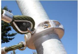
Corocord aluminum clamps are used as connectors between steel posts and rope. Two aluminium castings are bolted together. The height of the clamps is thus variable.
