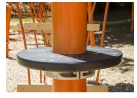
Discs are made of highly durable, eco-friendly HDPE, which is not only recyclable after use, but also consists of a core produced from 100% recycled material.
