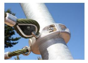
Corocord aluminum clamps are used as connectors between steel posts and rope. Two aluminum castings are bolted together. The height of the clamps is thus variable.
