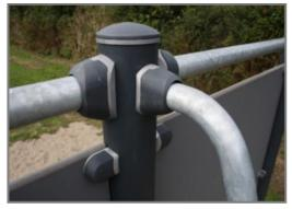
The connectors are made of die-cast aluminum, specially alloyed for the outdoor environments and heavy usage. The screws attaching the connectors are stainless steel and protected by zinc washers
