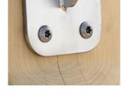
Stainless steel screws and/or screws covered with plastic caps,
