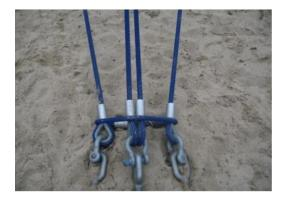
Huge spacenet structures are secured to the foundation with a system of three turnbuckles. Horizontal and vertical edge cables are fixed to individual turnbuckels, wich then connect to individual steel anchors. This system ensures that each edge cable can be tensioned separately and increases structural safety by way of independent anchoring.
